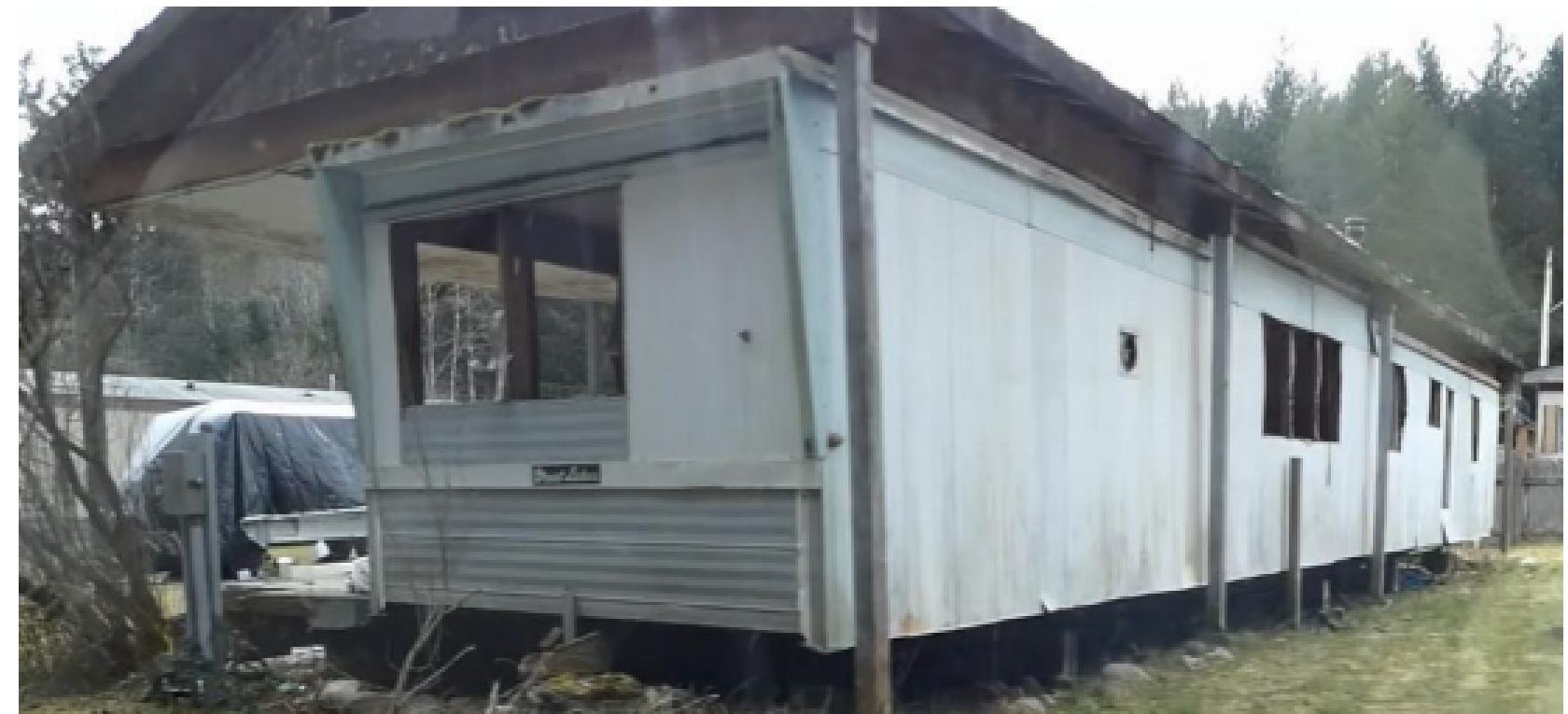
Building condition in Mobile Home Park
